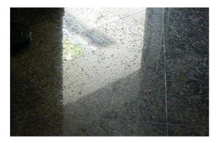
b. *Fissures:* The term "fissure" is used in the stone industry to describe a visible separation along inter-crystalline boundaries. This natural separation may start and stop within the face of the stone or extend through an edge. A fissure differs from a crack in that it is a naturally occurring feature of the stone. Once installed, fissures do not pose any structural issues.
